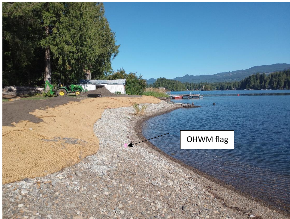
Photo 4: Bulkhead removal, shoreline restoration and OHWM identification.
